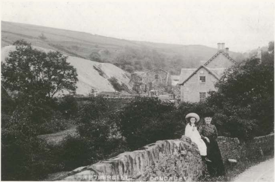
Nethergill. The ruins of the lead smelt mill can be seen to the left of the former mine offices. Mrs Gill and her daughter Elise lived at Hadfield Cottage which is just out of the picture on the right. (Photo. early 20th c.)
