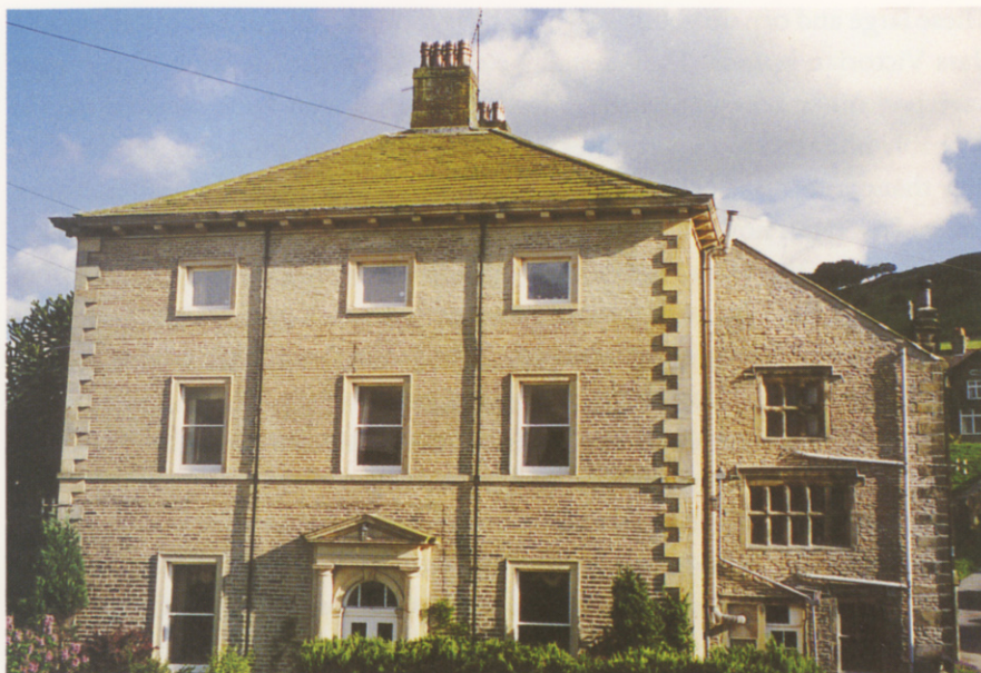
Cononley Hall. There is a distinct difference in style between the remaining wing of the 17th century Hall and the 18th century Hall on the left of this view.
