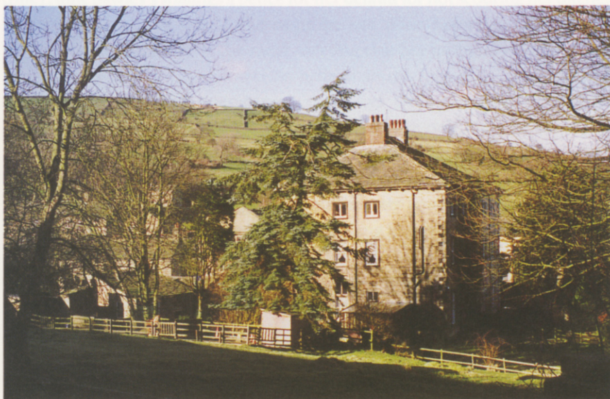
Cononley Hall from the south. The formal gardens of the Hall have now disappeared but were once to be found on this side of the building.
