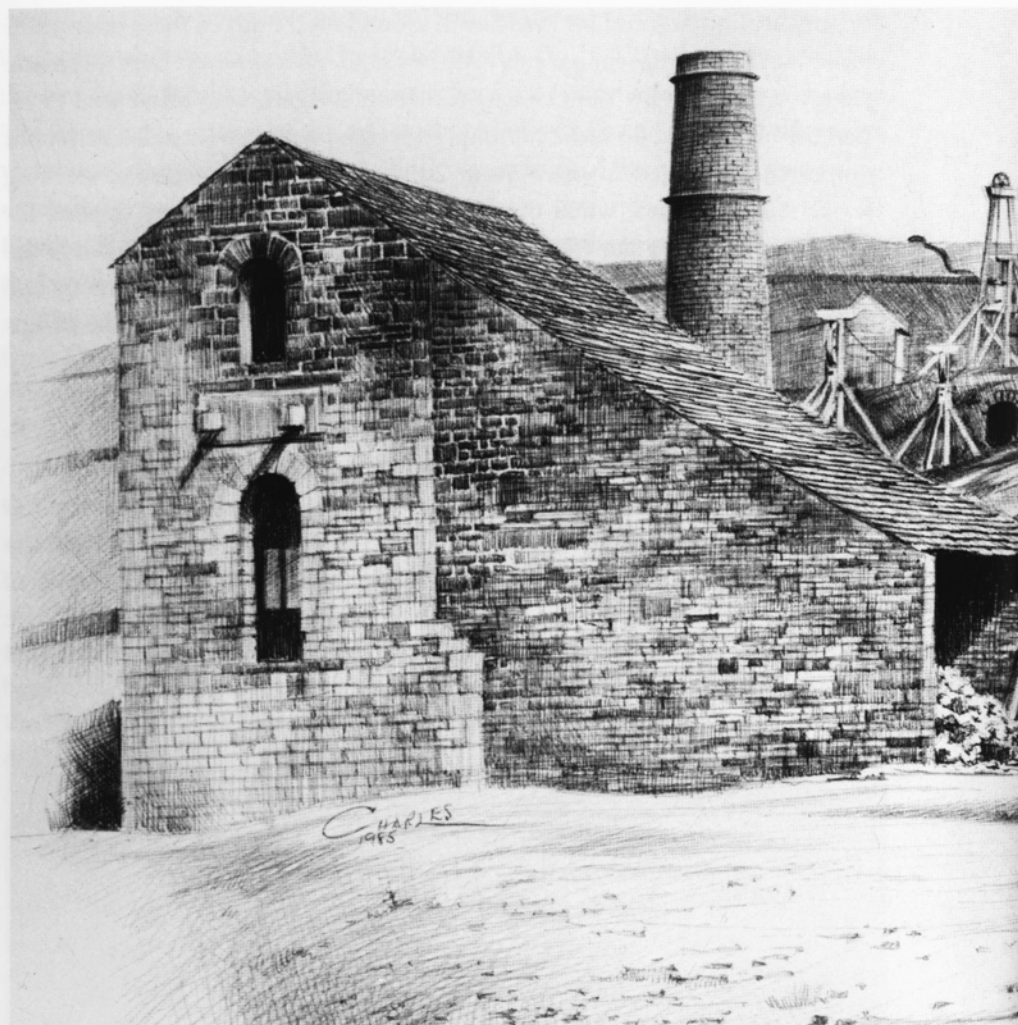
A reconstruction, based on photographic evidence, of the Lead Mine as it might have appeared at the time of its closure.
