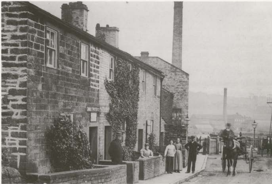
Main Street. Cononley's Postmaster, Peter Nelson, stands by the Post Office door. Also visible is the end wall and roofline of the mill, which were subsequently altered. (Photo. early 20th c.)
