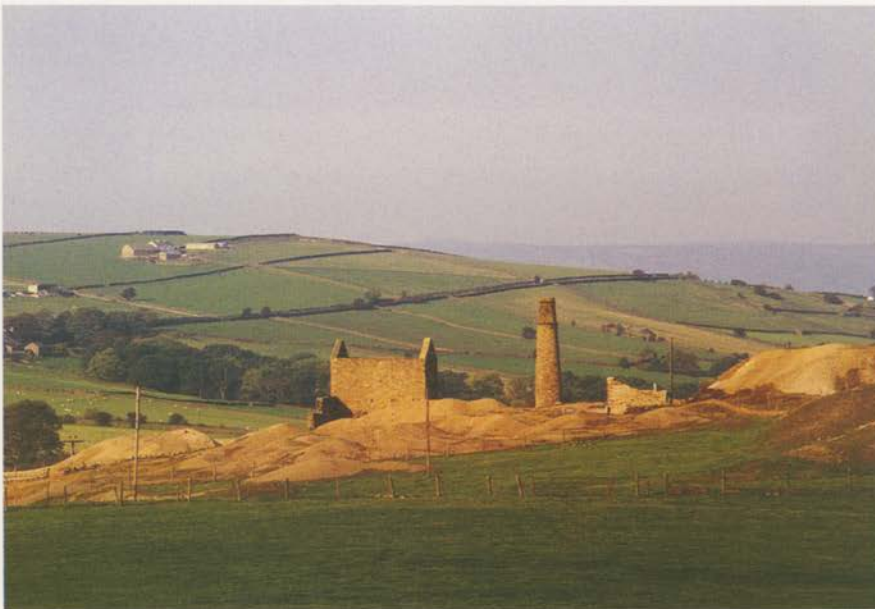
The ruins of Cononley Lead Mine engine house and chimney seen from the south.
