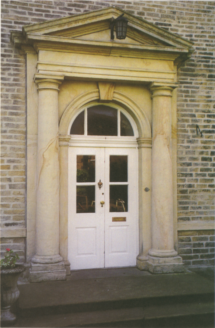
Main entrance to Cononley Hall.
