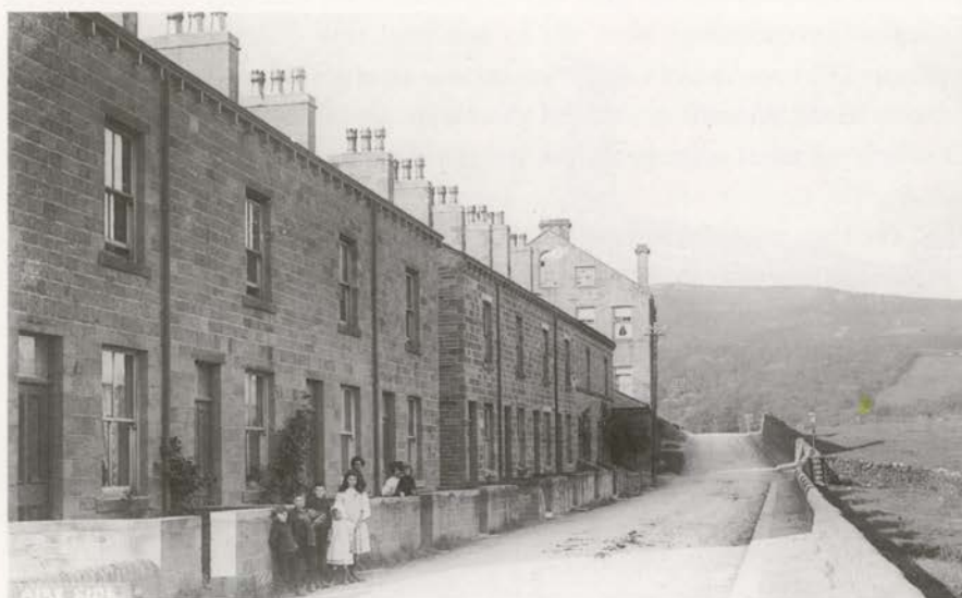
Aireside. The terrace must be almost new in this view although the two houses furthest from the camera are somewhat older. The visible part of the mill was also occupied as a house by its manager. (Photo. early 20th c.)
