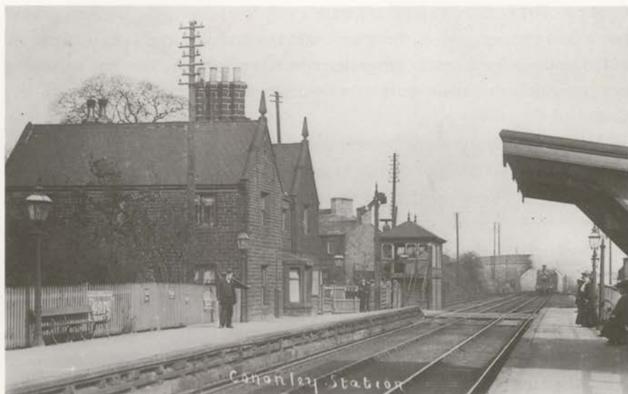
Cononley Station. A Midland Railway train is approaching the platform. (Photo. early 20th c.)
